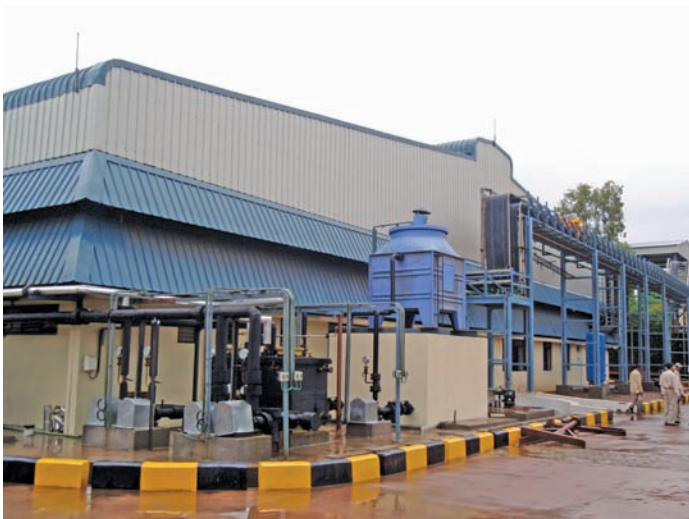
Water Based facility at Lote Plant
